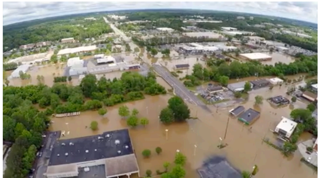
Drone pilot Mark Turner captured video of widespread flooding along Crabtree Creek in the area of Wake Forest and Six Forks Roads in Raleigh in April 2017. BY MARK TURNER
