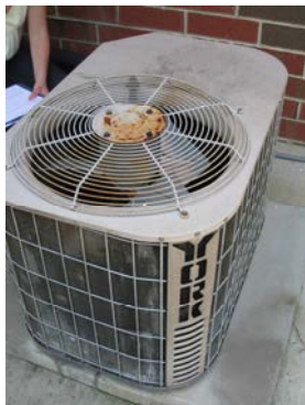
York 3.5 ton 10 SEER unit at Station 21 Carrier 3.5 ton 10 SEER unit at Station 6
