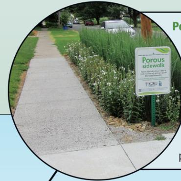
**Bioretention** located in the right-of-way can treat runoff from the street or rooftops where pollutants build up and then wash off between rain events. They can also shade the adjacent roadway and beautify the streetscape.
