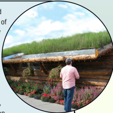
**Bioretention areas**, or rain gardens, are engineered landscape features that reduce runoff volume and pollution by capturing and temporarily storing or infiltrating runoff through soil, stone, and vegetation. They can also provide bird and insect habitat and improved aesthetics.
