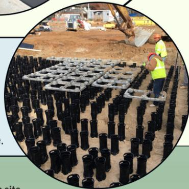
**Pervious plazas.** Incorporating permeable pavement in plazas, sidewalks, or open space area can reduce impervious area and provide additional opportunities for treatment and infiltrating of stormwater runoff.
