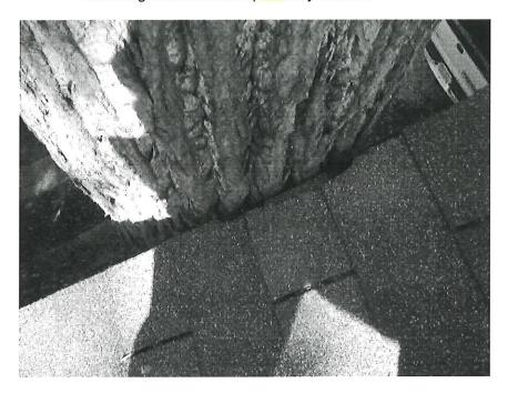
**Minor Repair** 4 Significant debris and branches need to be removed from the roof and the gutters need to be cleaned.
