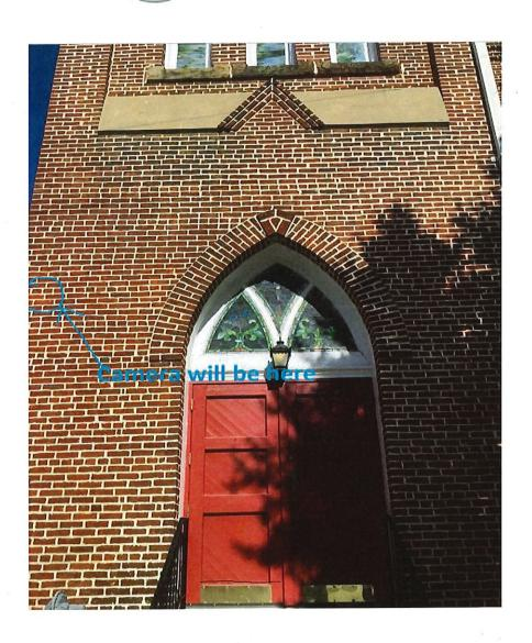
Front-right of church (W Edenton Street)- Dome camera will be mounted at front right edge of building and higher than door where shown below. Wires will be run from inside building and penetrate thru wall. Approximately 3-5 inches of conduit (painted to blend with wall) will be run and tied into mortar joints.
