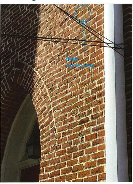
Front-left of church (W Edenton Street)- Dome camera will be mounted at front left edge of building and higher than door where shown below. Wires will be run from inside building and penetrate thru wall. Wires will not run on outside of building.
