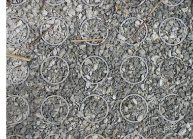
Photo 36. Close-up of vertical drainage pipes in crushed stone.
