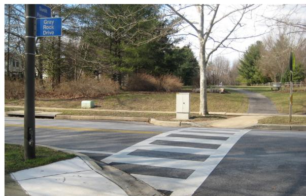
Photo 31. High visibility crosswalk with parallel bar.
