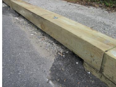
Photo 35. Close-up of timber curb raised to allow for drainage.
