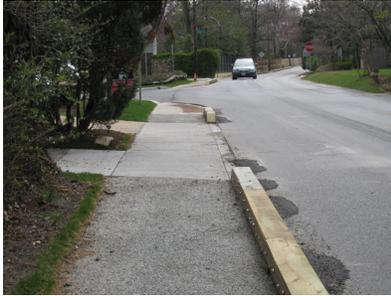
Photo 34. View of crushed stone sidewalk with timber curb.
